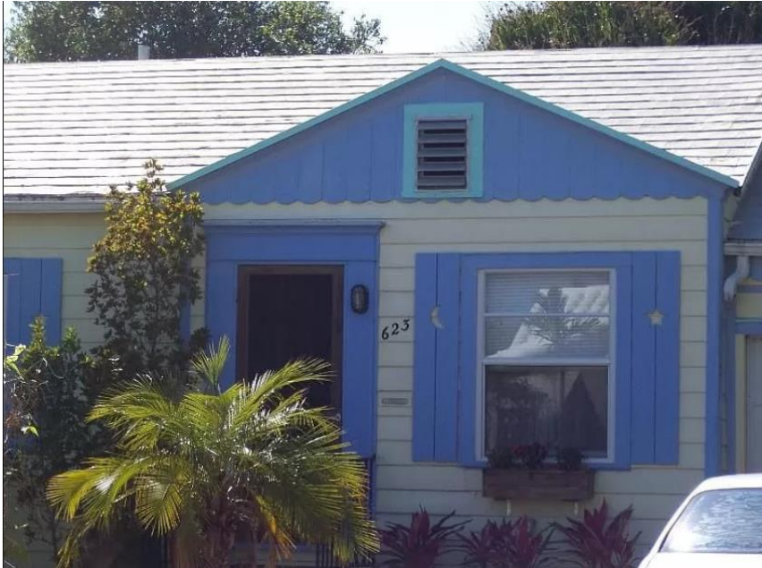
Image of the existing roofing system.
